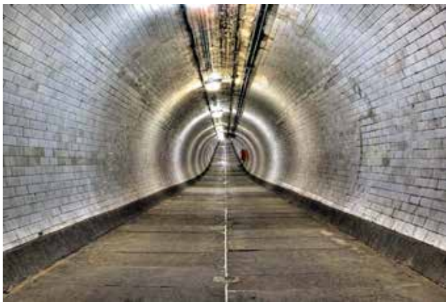
Before refurbishment the Greenwich tunnel was also grubby and unwelcoming
